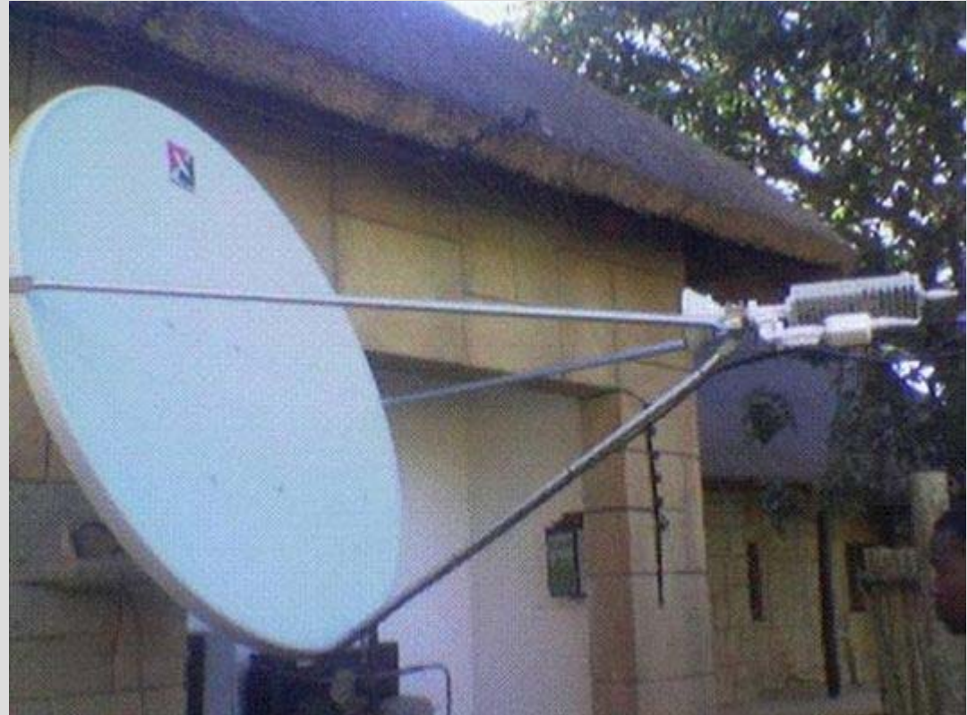
Channel master Ku band VSAT dish
