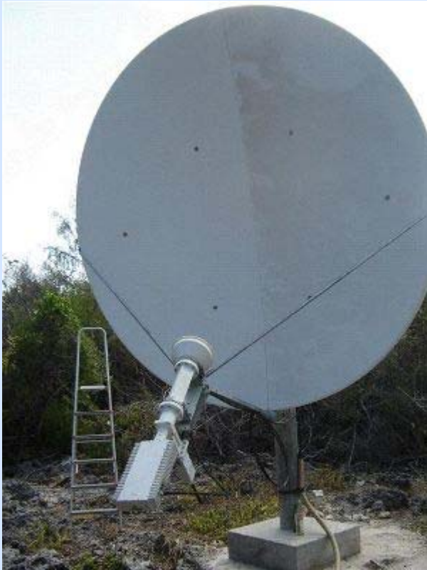
C-band circular polarization VSAT dish
